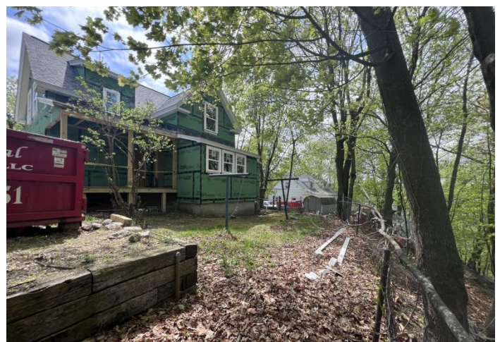
Construction Progress Spring 2025
